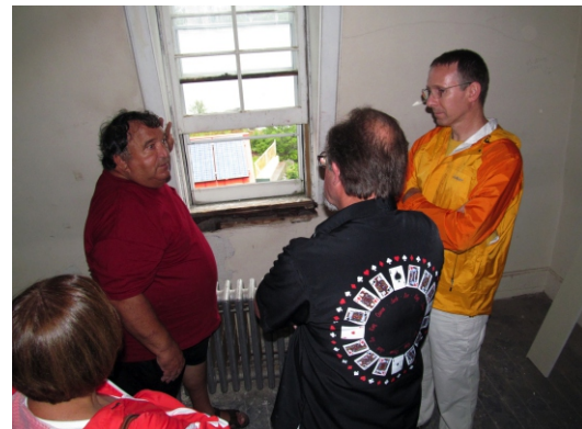
by Bob Trapani Joe Estrella showing members damage from leaking windows
