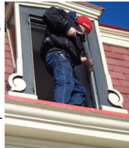
Putting in new storm windows
