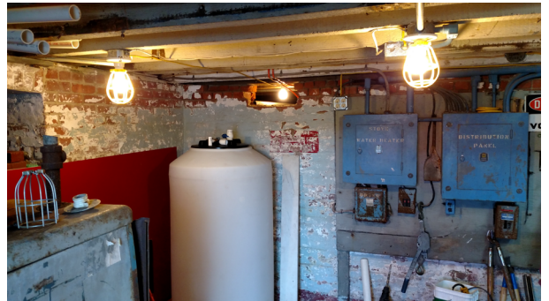
Joe and Dennis have installed lights themselves in the cellar
