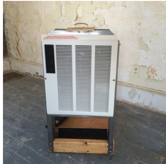
One of the 4,000 watt, 220 volt electric heaters
