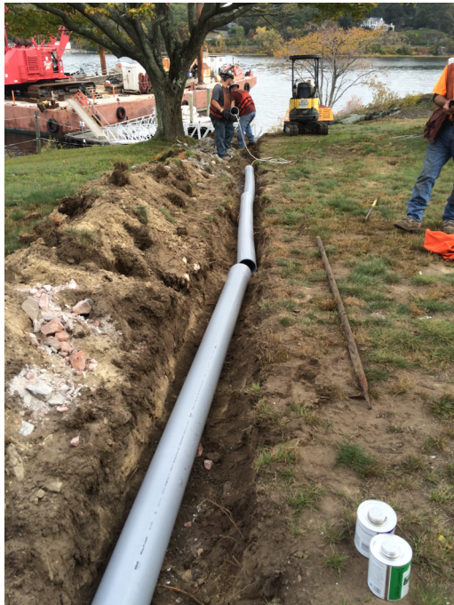
Cable laying on the island
