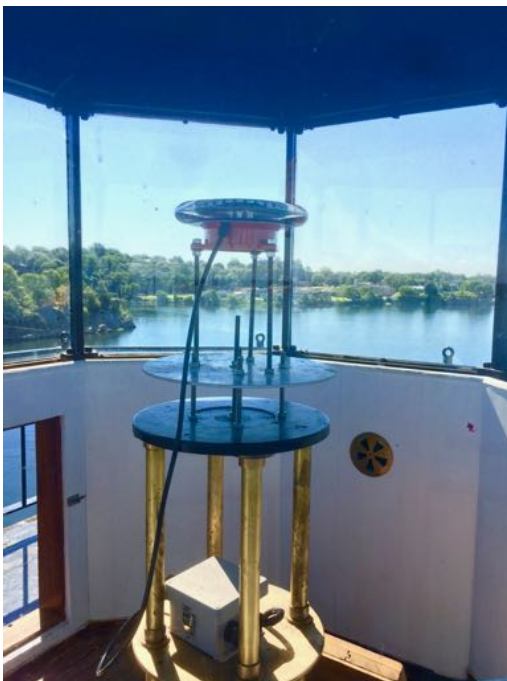
The new LED Marine Beacon now in use at Pomham Rocks Lighthouse
