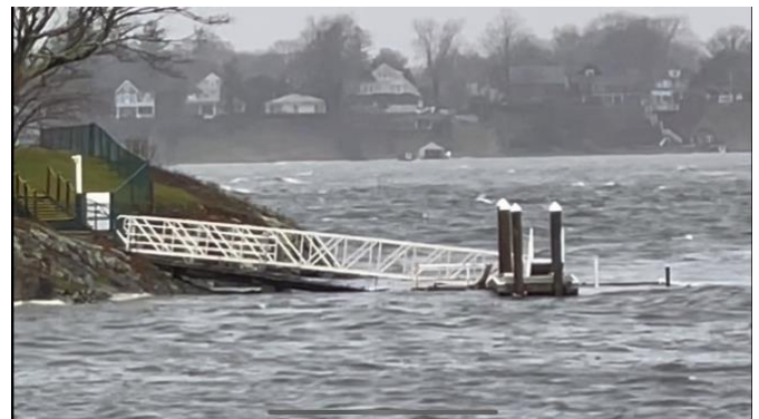
Dock Submerged by Storm Surge
