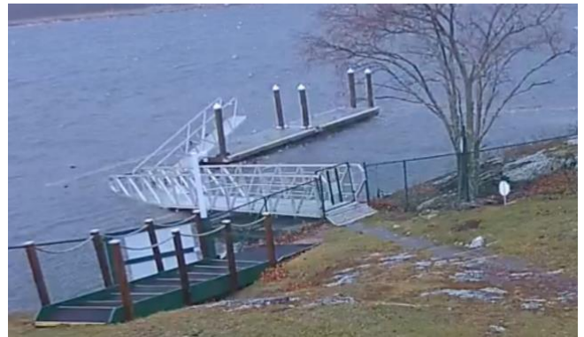
Security Camera Photo of Dock Submerged
