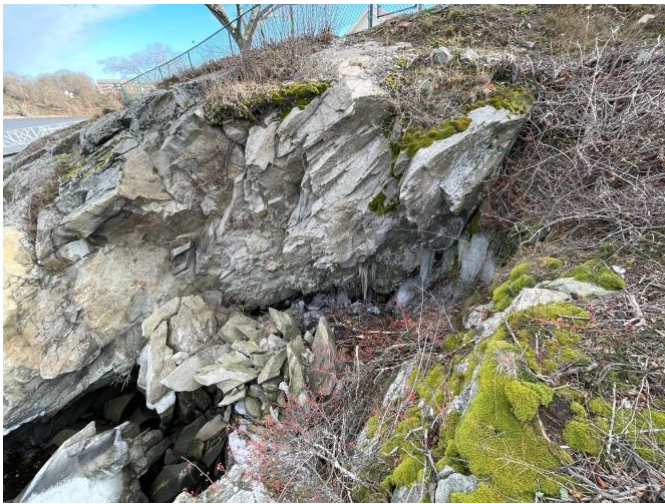
Collapsed Section of Ledge
