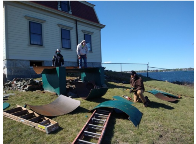
Oil Tank Removal
