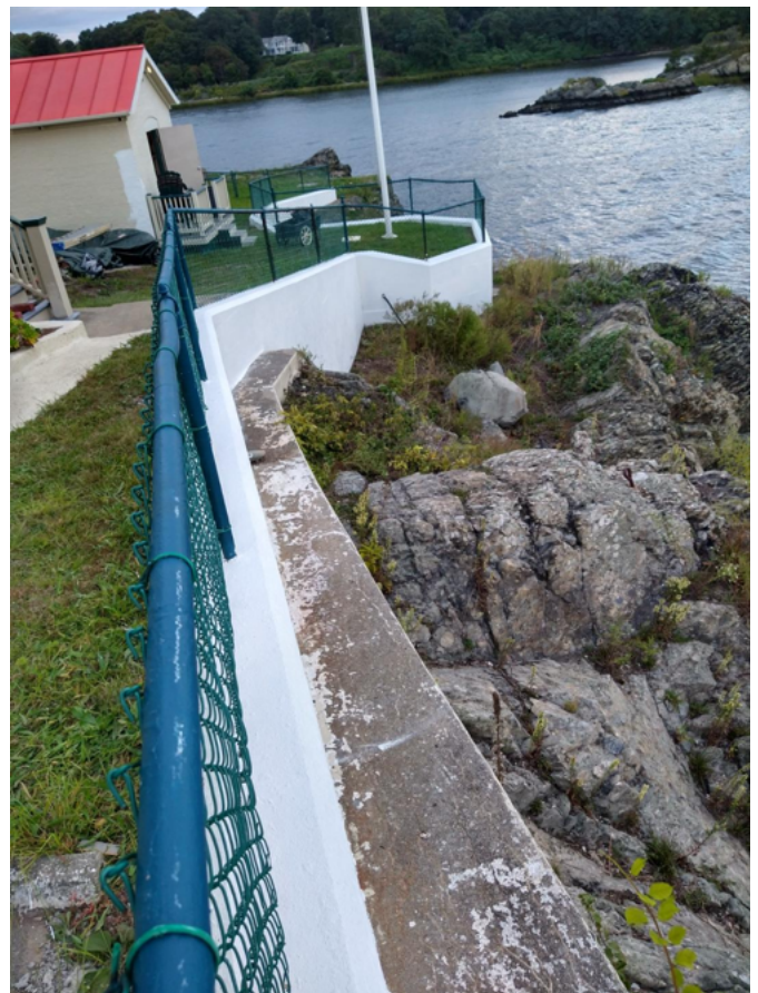
Freshly painted south retaining wall
