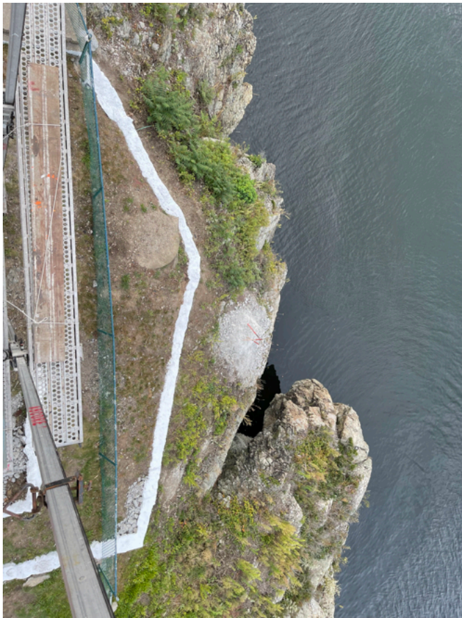
View of stone wall from lantern room
