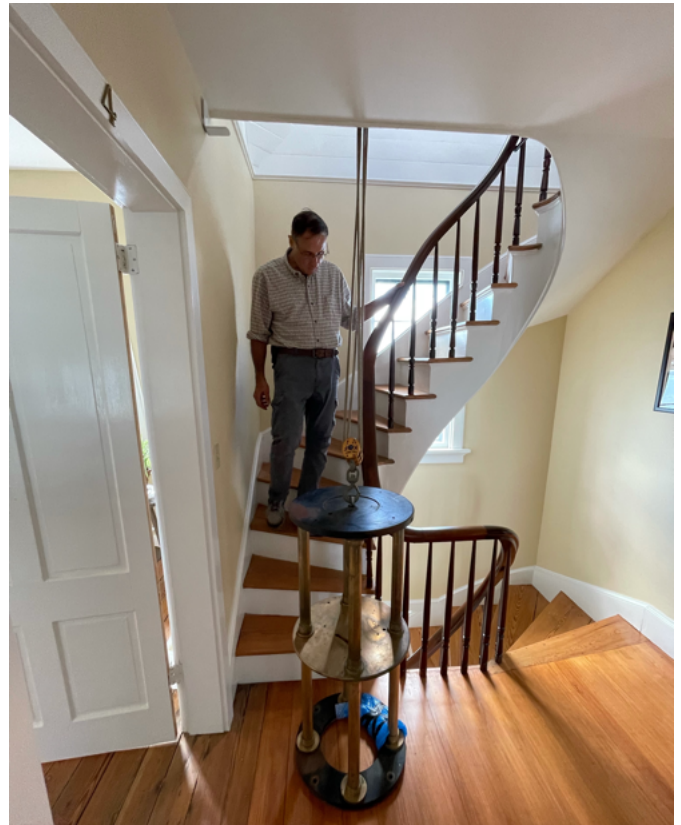
The original 4 th order pedestal being lowered from the lantern room by block and tackle
