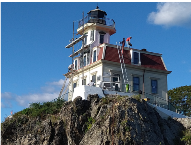
Wood rot replacement nearly complete
