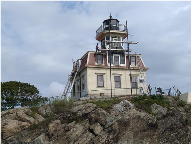
Watch room being sealed with weather wrap, trim to be added.
