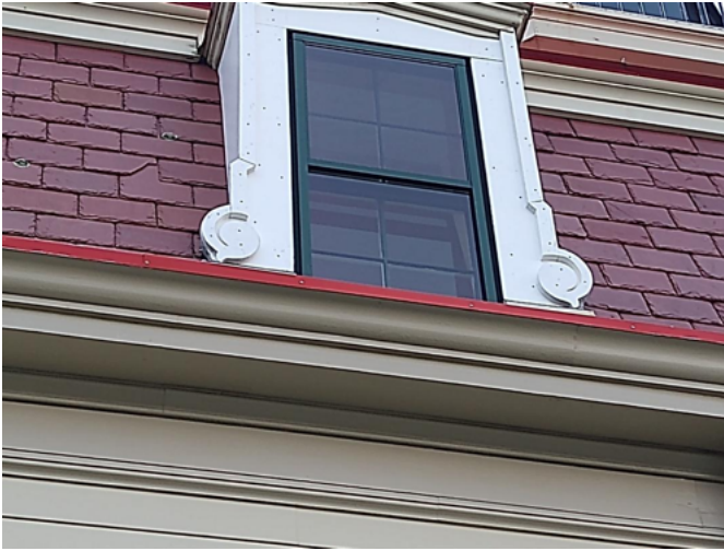
Replaced window dormers and trim
