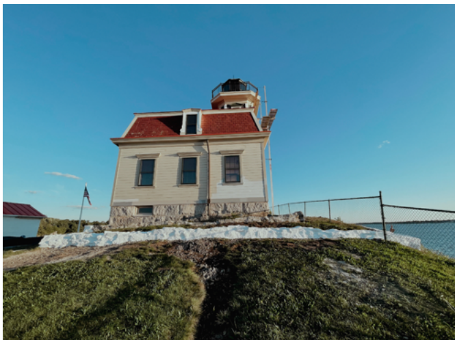
Stone wall almost complete
